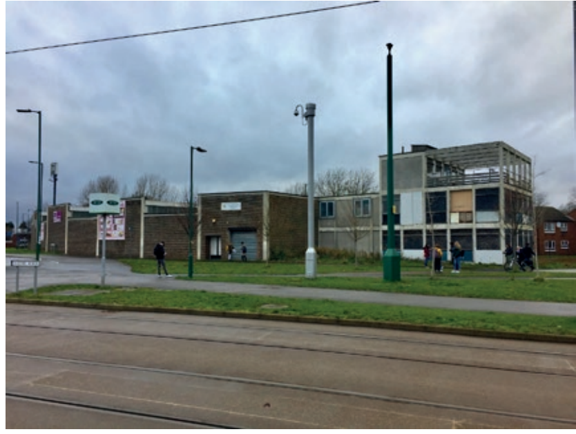
Shown above is the appearance of the original building as seen from the nearest tram stop.
