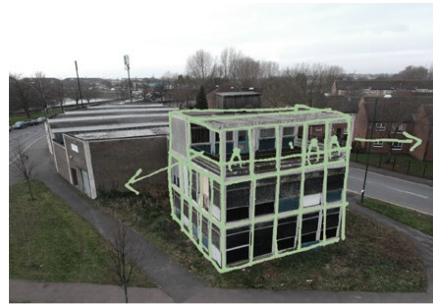
Views out over the city from roof terrace in the cube
