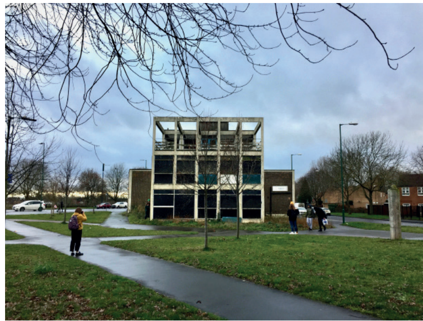
We felt that the proportions and layout of the administrative end of the warehouse were interesting and identified this as something to carry into the future design.
