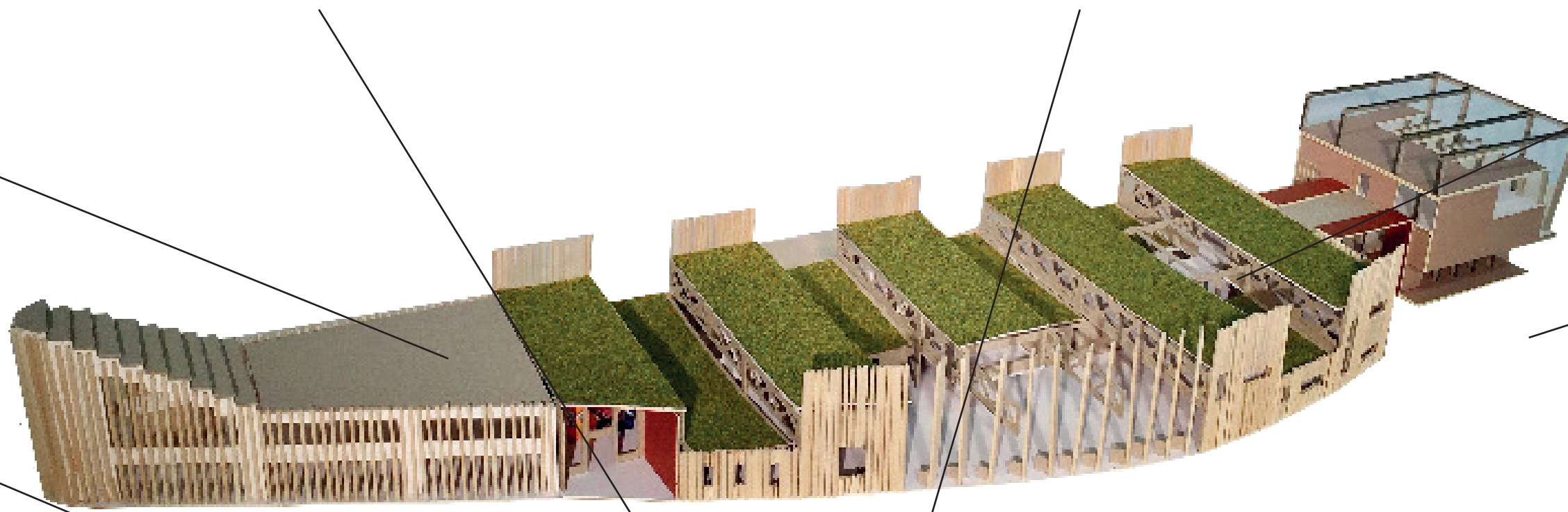
The wood cladding, that runs across the whole main section of the building is manipulated to create openings for windows and views into and out of the large void which is used as an exterior extension of the daycare.
