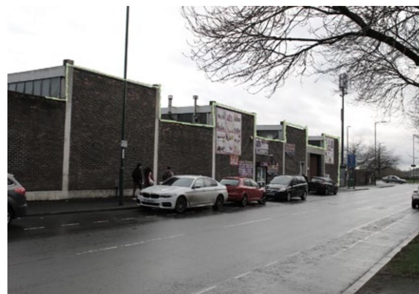
Repetitive roof line
