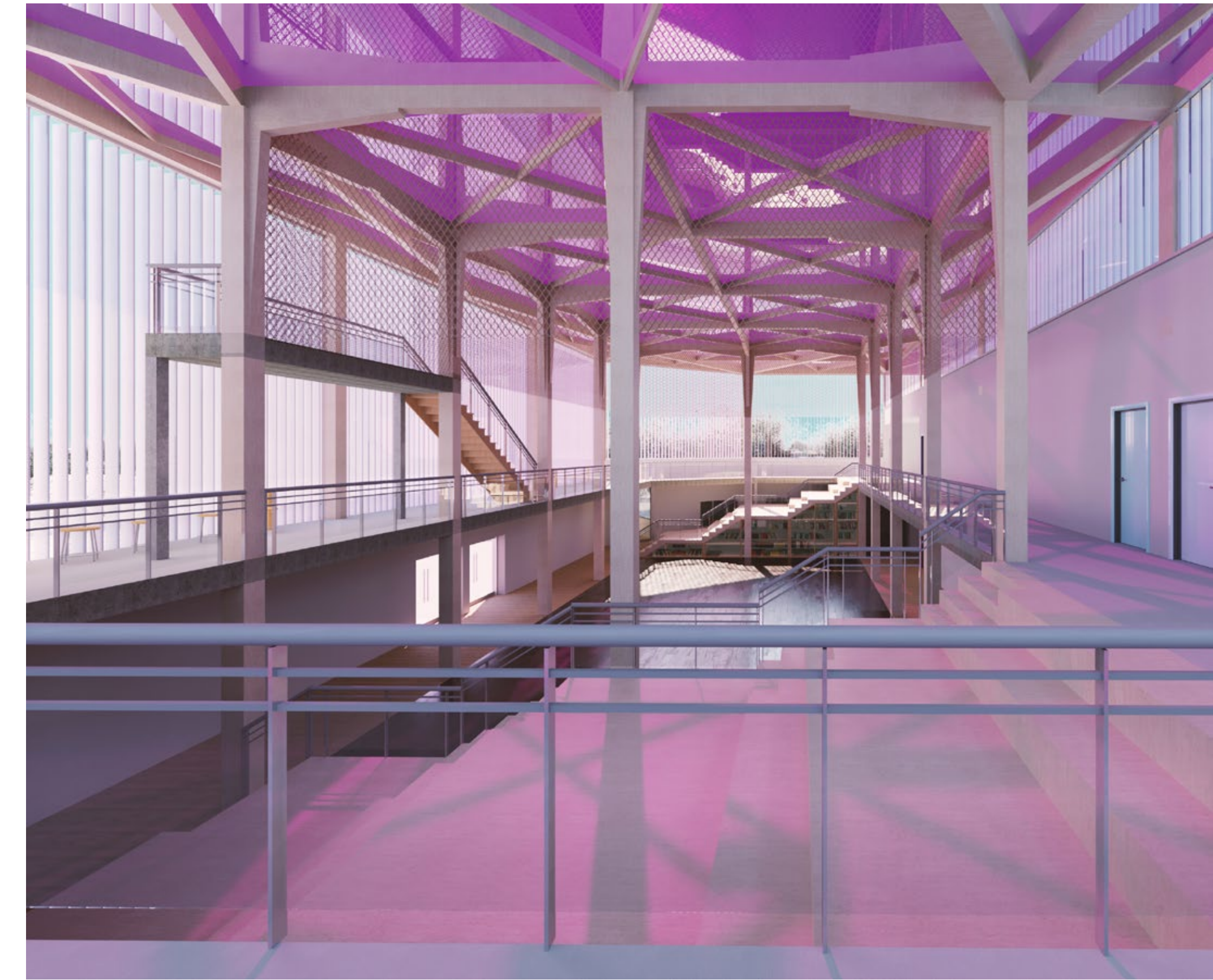
Glazed roof transitions to a deep purple to stop solar gain
