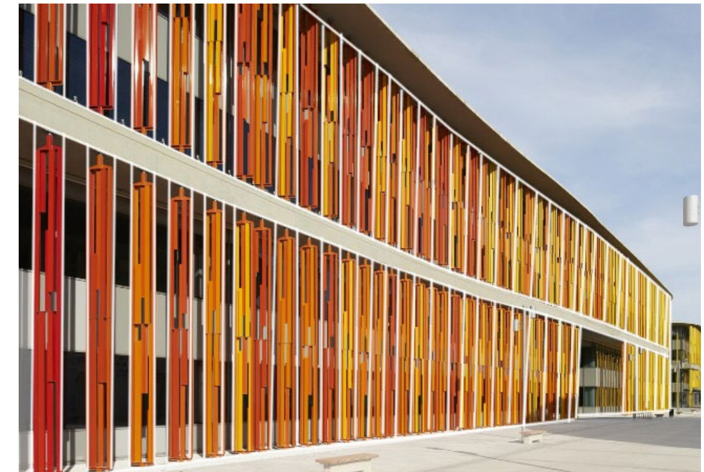
The Ronda Building - Estudio Lamela External horizontal fins change colour from deep red to yellow, help inhibit direct solar gain.
